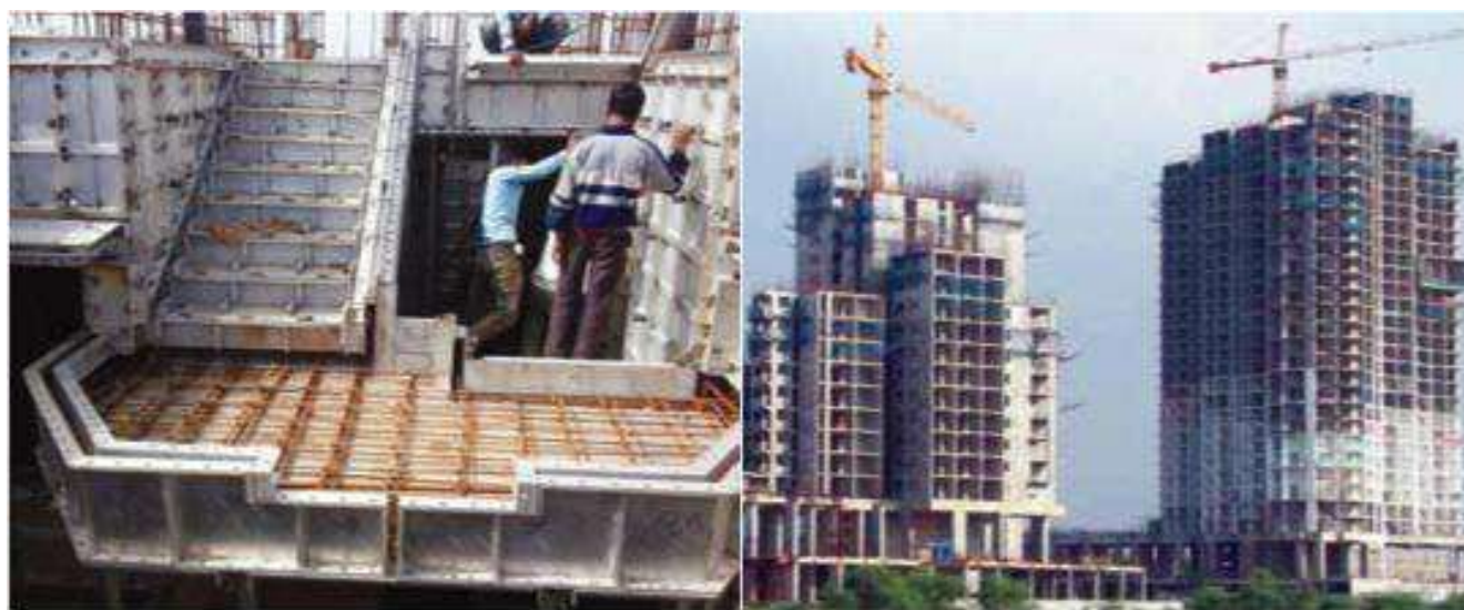
Figure 32: Monolithic concrete construction using aluminum formwork
