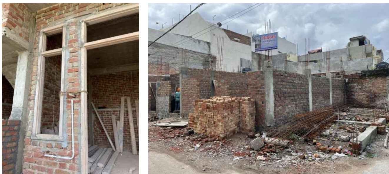
Figure 36: Red brick construction is the norm in Jaipur (left) and Indore (right)
