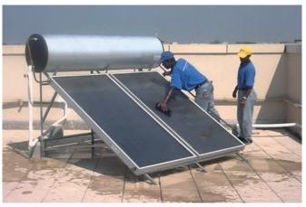
**2.** Roof is recommended for installation. The collectors should face South direction for maximum sunlight.
